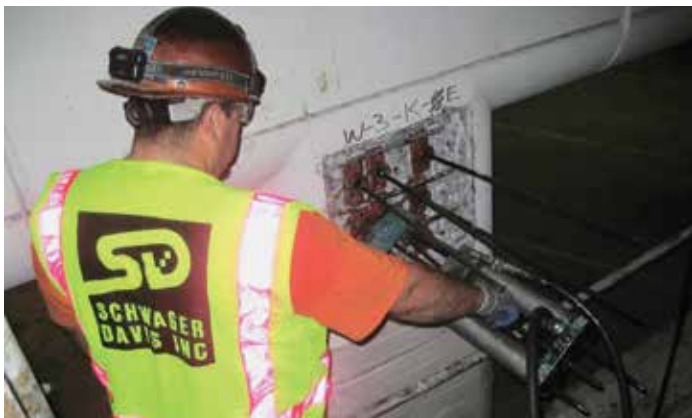
Figure 4. Worker re-tensions a repaired strand.
