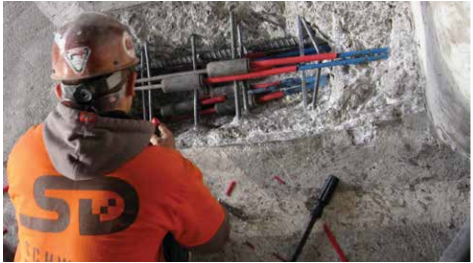
Figure 1. Worker repairs parking garage slab PT strand with couplers.
