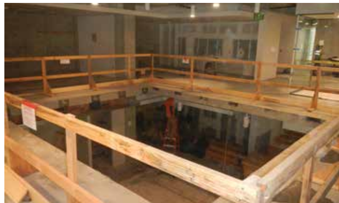
Figure 5. A successful PT slab cutout for a new staircase.
