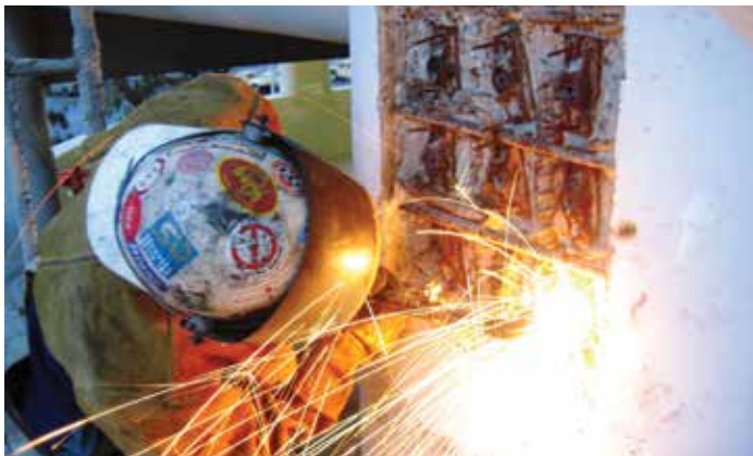
Figure 2. PT worker detensioning a tendon to prepare for strand replacement.
